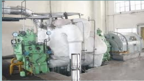
Direct Condensing Low Pressure Turbine Generator
